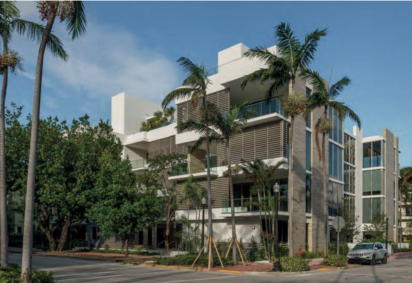
Louver House, Miami USA
