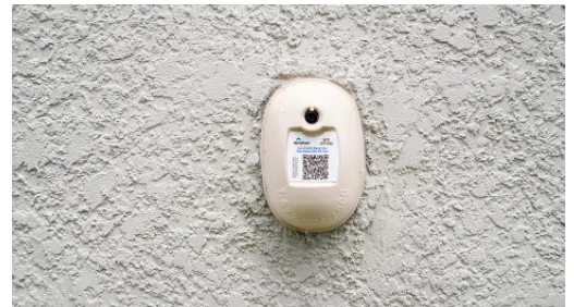
Built-in Taexx pest control system
