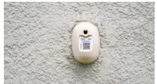
Built-in Taexx pest control system
